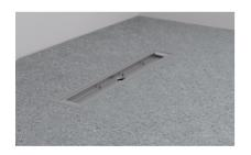
3. Fill the space under and around the channel with screed or a similar product to the level of the flange. Create a fall to the vinyl drain from all four sides.
