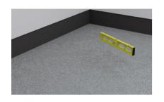
1. Set the level of the finished shower floor surface and mark it on the wall in the area where the channel will be fitted (allow for the slope of the shower surface).
