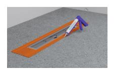
4. Use Superfix glue to seal surface around the drain. Superfix is a silyl modified polymer (SMP) based adhesive with a high tensile strength. Use a glue gun to better distribute the substance.
