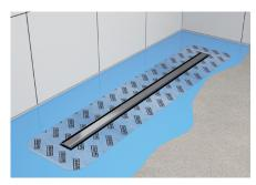
5. Unfold the membrane and slightly press it to the wet foil to ensure close adherence.
