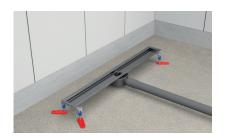
2. Connect the linear drain to the plumbing system. Set the height of the frame taking into account the thickness of the tiles. Set the height using the adjustable legs (optional additional payment) so that the upper edge of the frame is app. 1mm below the height of the tiles.
