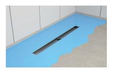
4. Cover the flange and the surrouding area with an insulating foil in a liquid form.
