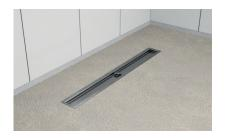
3. Fold up the membrane to keep it clean. Fill the space under and around the linear drain with concrete/screed to the level of the flange with the correct slope.
