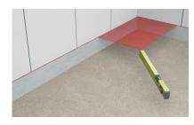
1. Set the level of the finished shower floor surface and mark it on the wall. Remember to allow for the slope to the drain.
