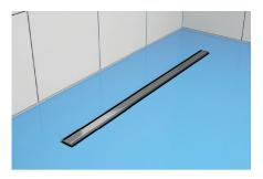
6. Apply a second coat of the liquid foil to whole surface of the shower area and sealing membrane.
