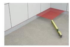
1. Set the level of the finished shower floor surface and mark it on the wall in the area where the channel will be fitted (allow for the slope of the shower surface).
