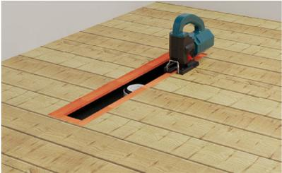
2. Use jig saw to cut across the previously marked linear drain shape. Remember to make an additional cut in the floor so that the linear drain flange is placed flush with the wooden floor.
