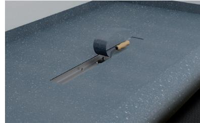
6. Roll out the vinyl flooring. Remember to install a vinyl floor at least 100 mm on the wall surface. Carefully cut a hole along the inside edge of the VF clamp drain (use heat gun to soften the vinyl).
