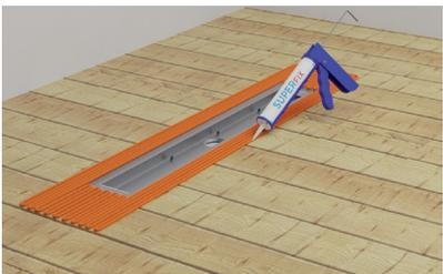
4. Use Superfix glue to seal surface around the drain. Superfix is a silyl modified polymer (SMP) based adhesive with a high tensile strength. Use a glue gun to better distribute the substance.
